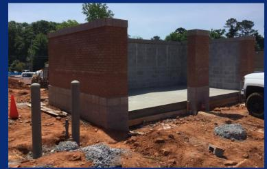
Dumpster pad brick complete and slab poured
