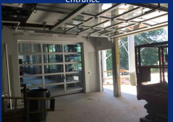
Overhead door installed in STEM lab
